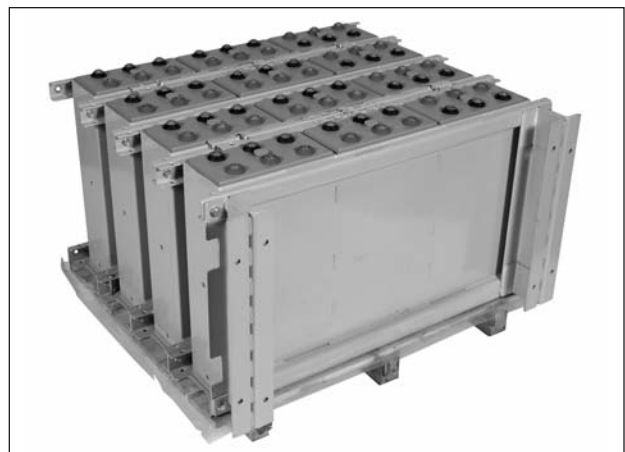
COMPLETED I-BEAM SUPPORT TO MODULE INSTALLATION Figure 10
