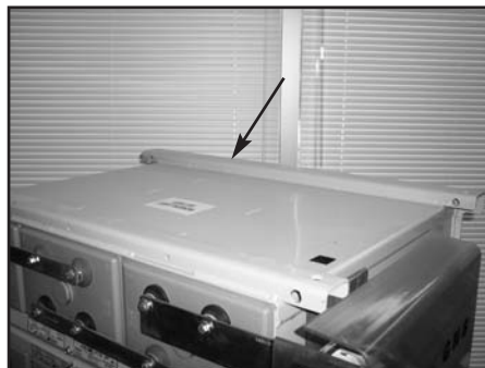
Figure 4: Recommended Frame Ground Location
