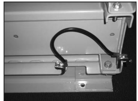
Figure 3: Cable Assembly Installation
